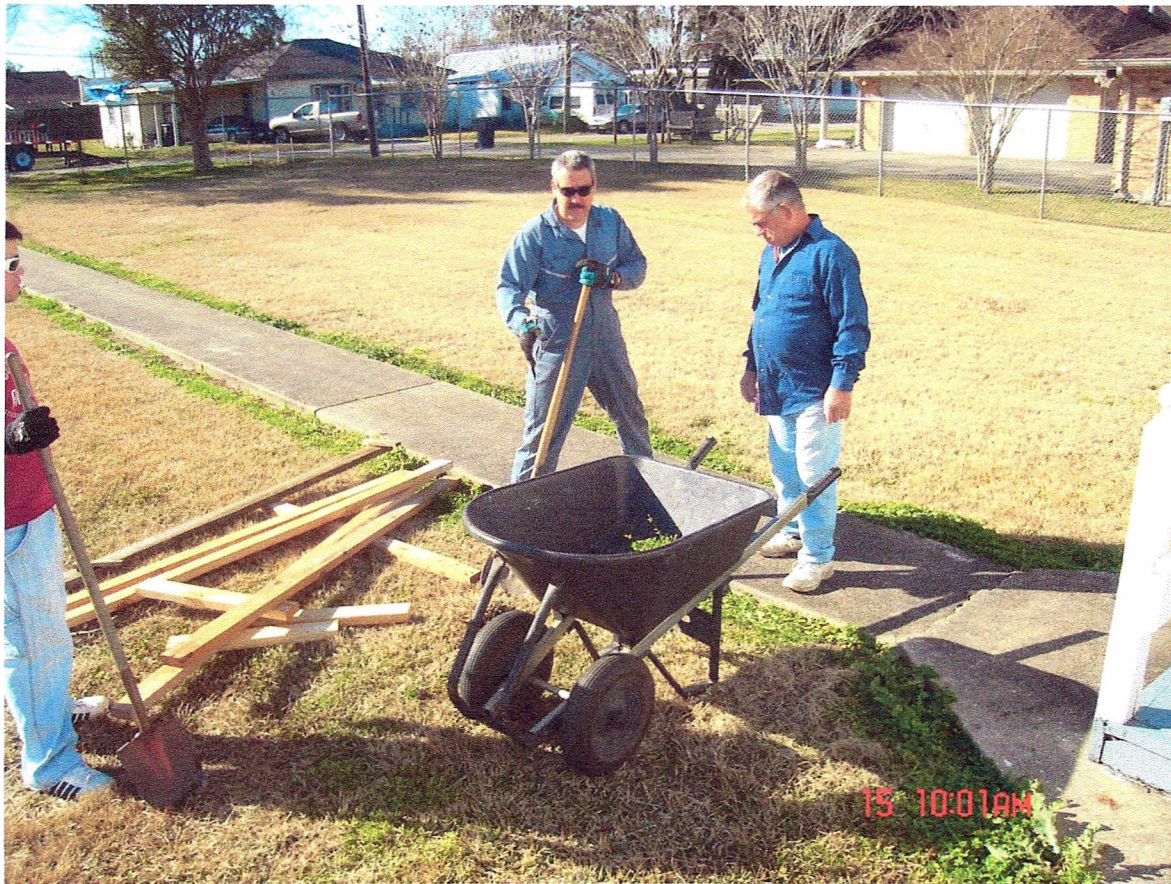
Cement slab work at the KC home. January, 2011
