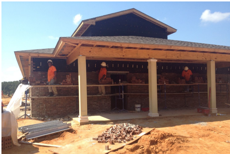
New St. Mary's Dormitory Under Construction
